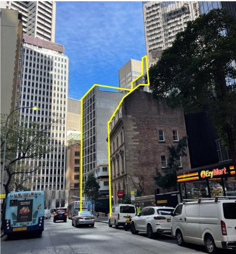
Figure 9. Eastern site, shown in yellow, viewed from Bligh Street looking south-west
